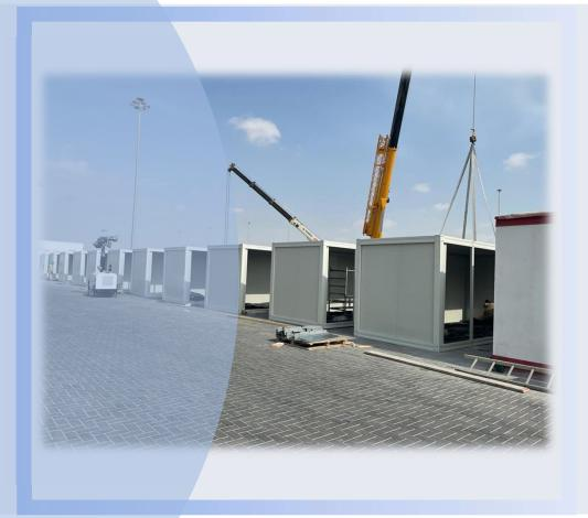
Bottom and Top chasis shipped as completed, only walls, doors and windows are needed to be installed at site.
