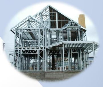
A new kind of living space is prepared by light steel structures. The system is based on galvanized unwelded steel technologies.
